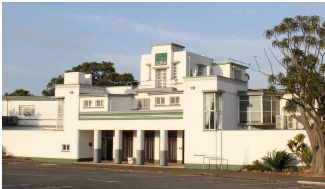
Stamford Hill Aerodrome Control Tower, Durban. Reproduced by permission of the SA National Society
