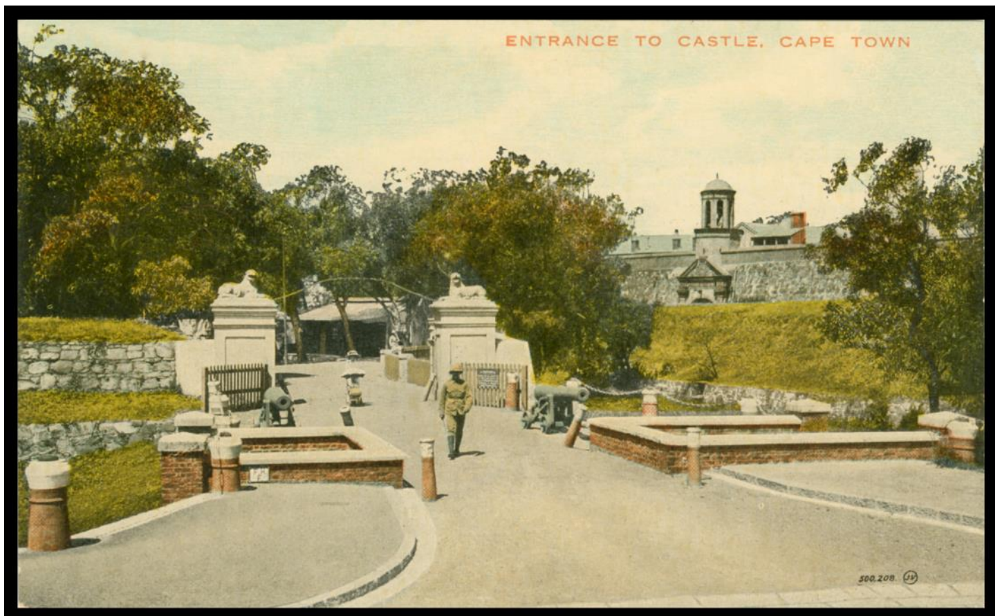
(Fig 2). The Castle, Cape Town: Built 1666 - 1679. Postcard. Circa 1910. Entrance to the Castle. (North facing). The Main Gateway is the pointed arch and look-out tower. The Outer Gate (with lions) seen from the eastern Grand Parade.
