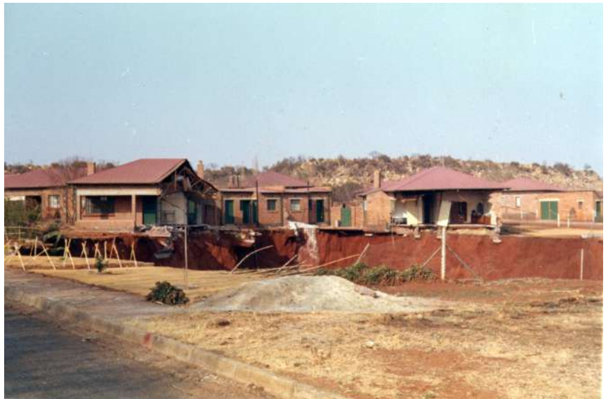
A picture of the subsidence of 3 houses in the suburb Westdene of Blyvooruitzicht Gold Mine in 1963
